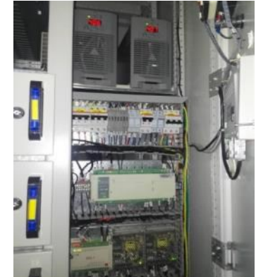
Converter and active protection equipment
